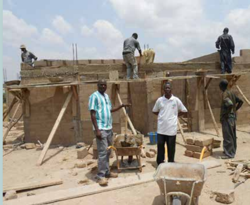
Brother Peter, clinic director, inspecting the construction progress.
